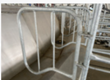
Head Dividers Prevents "feed robbing" between stalls
