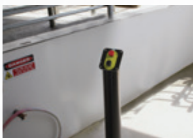
Platform Operator Console - E-Stop Can be activated in case of an emergency
