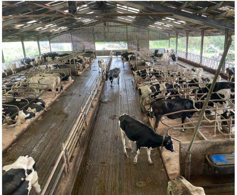
This shed has been totally refurbished. Improvements include new cubicles and waterbeds, the Feed Step and rubber matting on all passageways.
